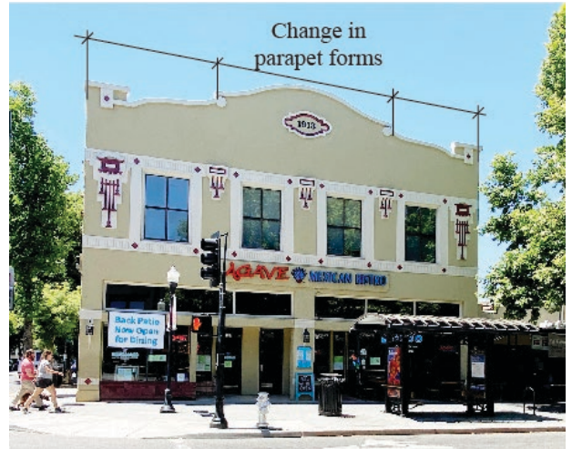
Fig. A.10: Interesting roof forms are encouraged throughout the downtown.
