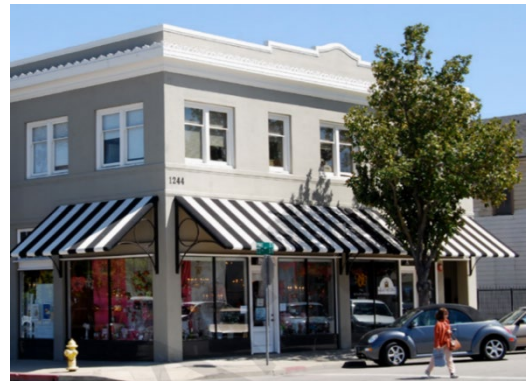
Fig. H.7: Canopies help provide a pedestrian scale to the building.
