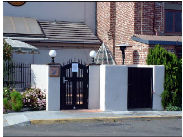
Fig. H.27: Trash and loading areas should be well screened from view in structures that are consistent with the building design in both materials and detailing.
