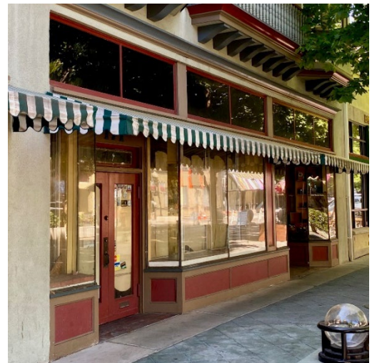
Fig. H.10: Entry alcove at street-facing building facade.
