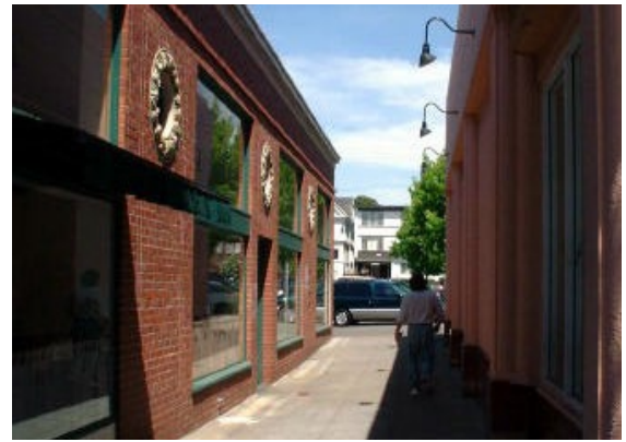
Fig. H.31: Pedestrian passageways leading from rear parking areas to Castro Street should be reinforced with features that provide interest such as windows, trellises, benches, planting, and attractive lighting.
