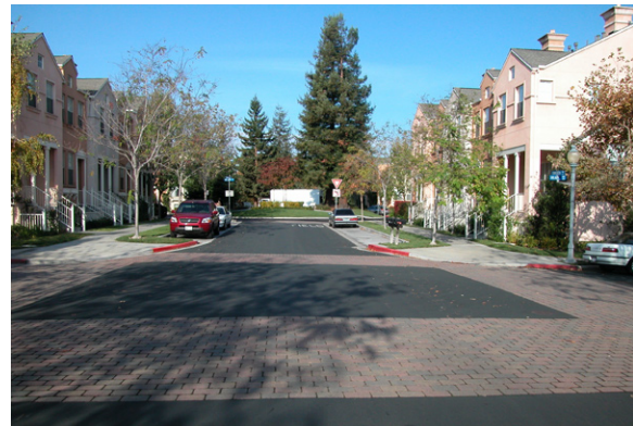
Strong crosswalks are created by a variety of details. Here special pavings are used to bring attention to the change in use and a mid-block bulb out to shorten the distance from sidewalk to sidewalk.
