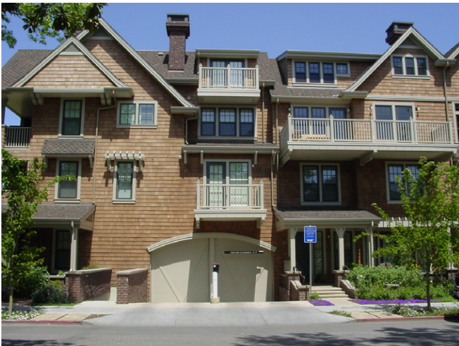
Entries to structured parking should be incorporated into building design and wrapped with habitable uses.
