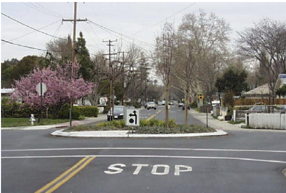
Small traffic circles at intersections slow down drivers and deter through traffic. (Farley Street, Mountain View)
