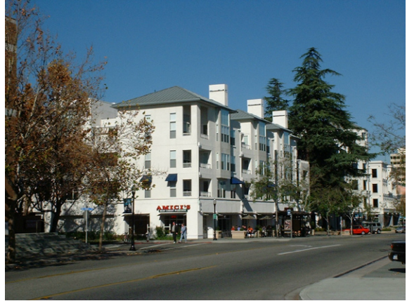
Example of a mixed-use corner retail building along Castro Street.
