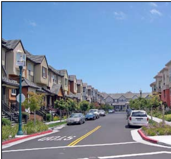
Bulb outs/neckdowns at intersections reduce the roadway width from curb to curb.
